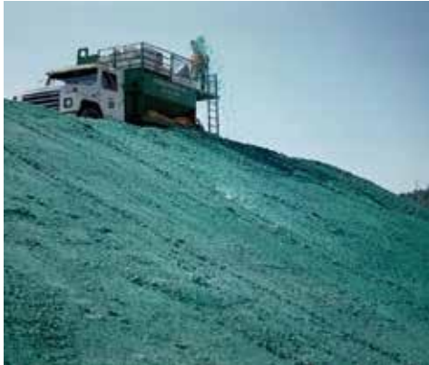
Forms an erosion-resistant blanket that prevents polymer leaching and dispersion of soil particles
