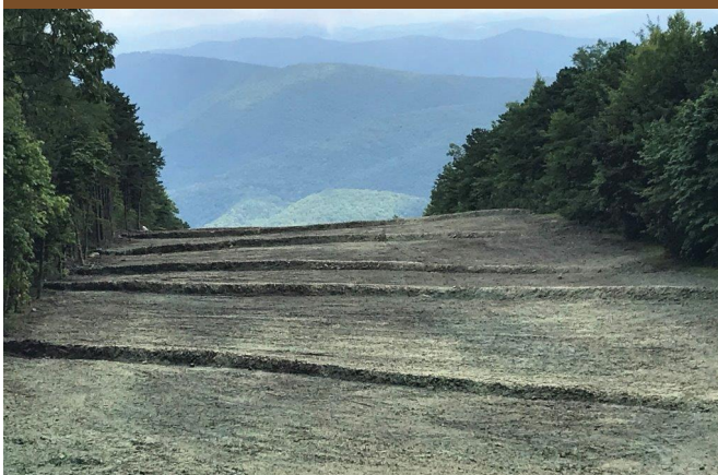
Energy / Pipeline Restoration
